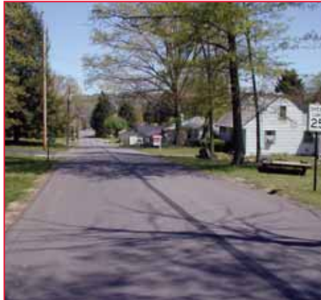
CDBG STREET IMPROVEMENT PROJECT
