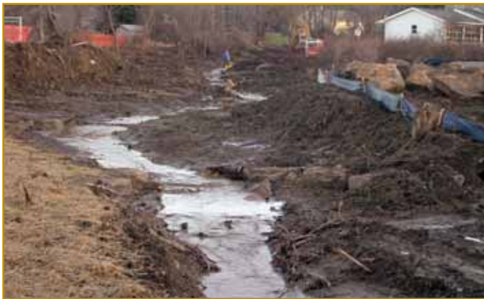
INDIAN RUN STREAM RESTORATION PROJECT
