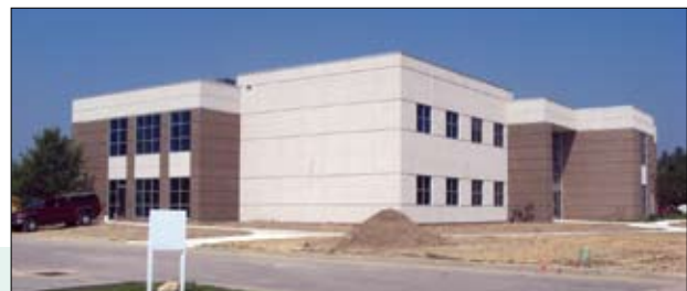
The Butler County Community College (BC3) 20,000 square foot facility at LindenPointe nears completion.
