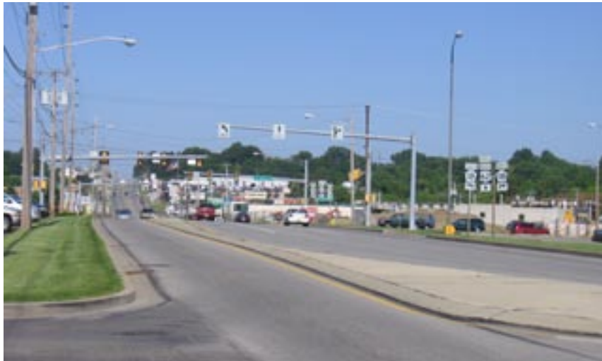
EAST STATE STREET LOOKING WEST TOWARDS INTERSECTION WITH HERMITAGE ROAD
